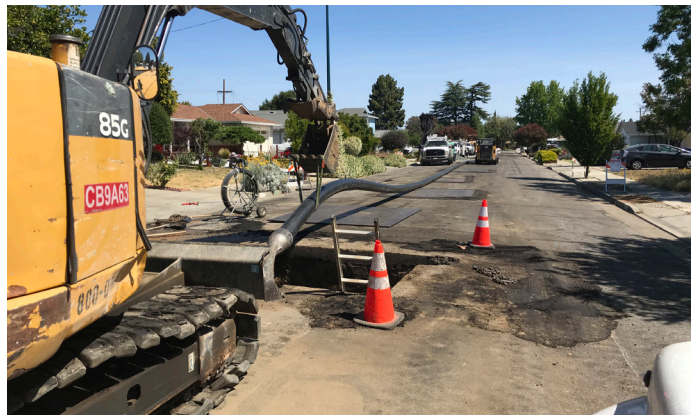
Figure 8. Pipe Bursting in Sunnyvale
