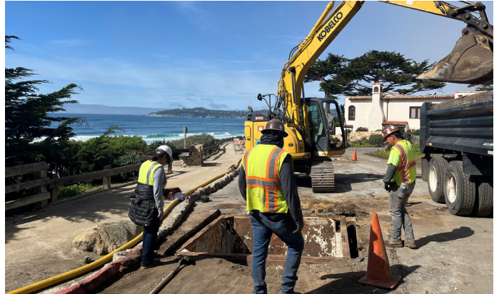
Figure 7. Pipe Bursting in Carmel
