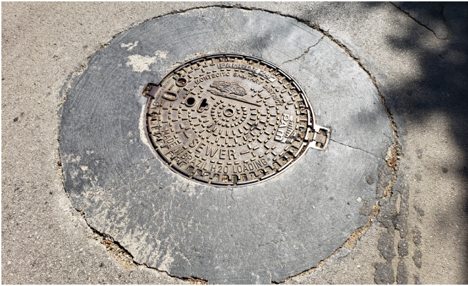
Figure 6. Existing Manhole in the Project Area
