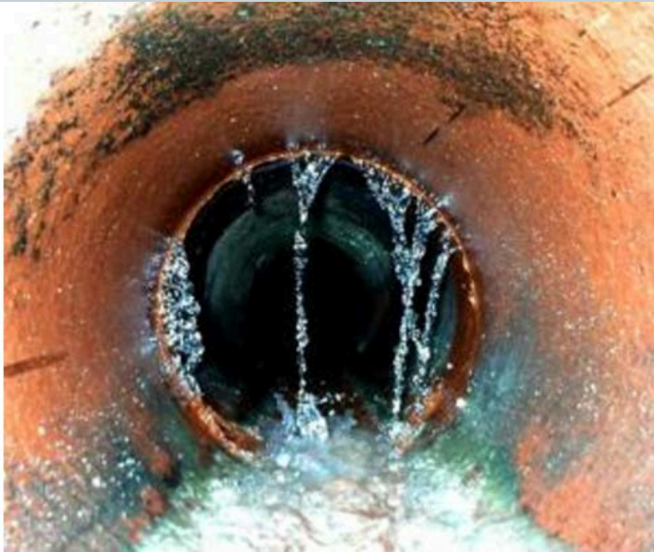
Figure 1: Sewer infiltration (Skipper, n.d.)
