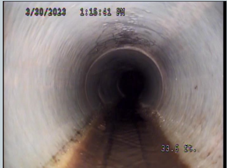
Figure 1: Sewer infiltration (Skipper, n.d.)
