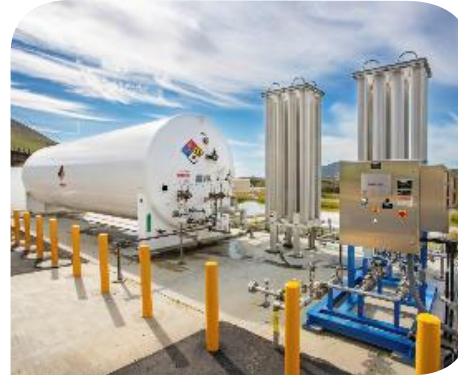
City of SLO WTP
